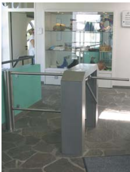
An automatic swing door beside the tripod barrier provides access for people with reduced mobility
